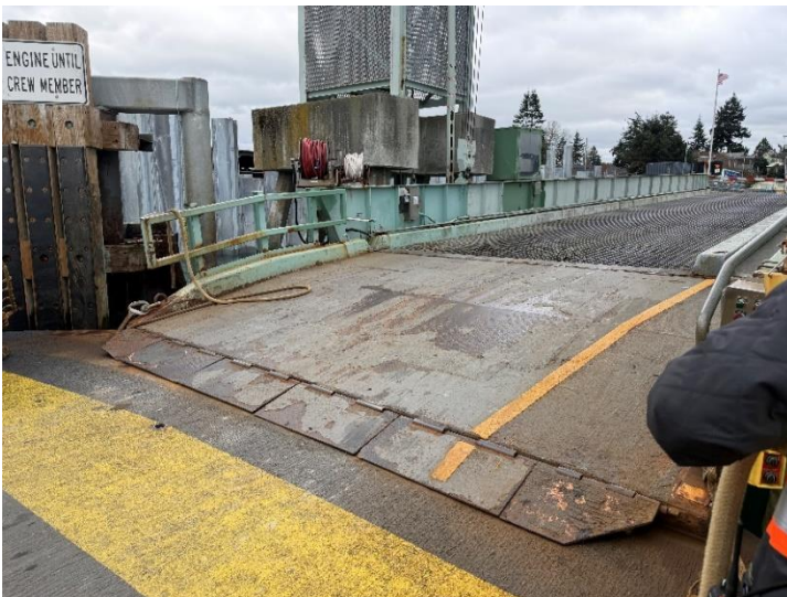
Anacortes Bridge Apron
